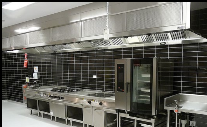
Campbelltown Hospital - Capturestream CS3
