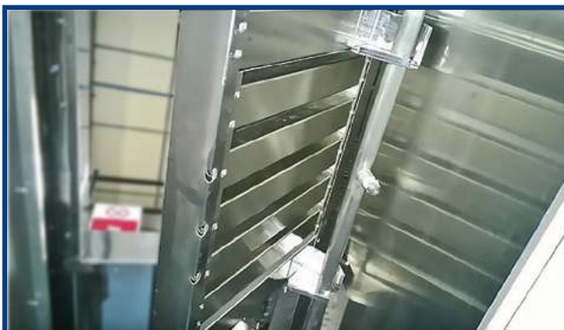
Britannia Filters and low consumption water mist nozzles
